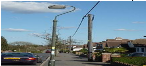
Figure 1: Example of an Insulated Bundle Electric Network
